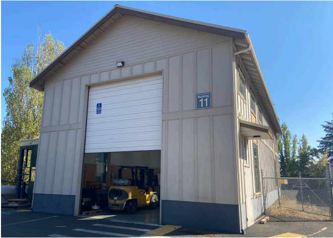
EXISTING BUILDING 11 EXTERIOR
